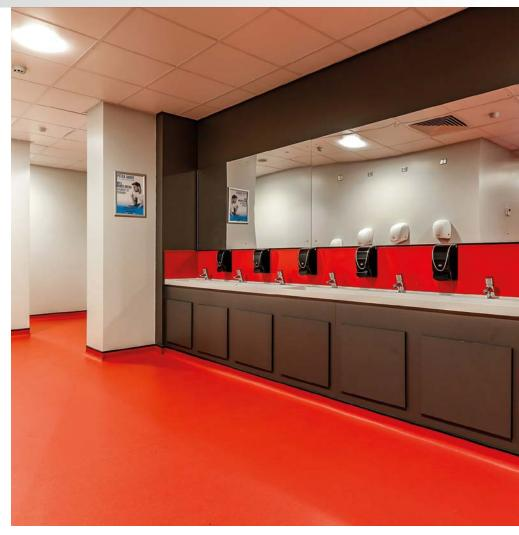
main contractor BAM Construction. As a result, just under 1000sqm of Gerflor's R10 slip-resistant Tarasafe Standard in colours, Poppy, Marbre, Noir and Storm were installed in the toilet and bar areas with 500 sqm of R12 slip-resistant Tarasafe Super in Dove Grey within the kitchen area, where a higher level of slip resistance was needed.
