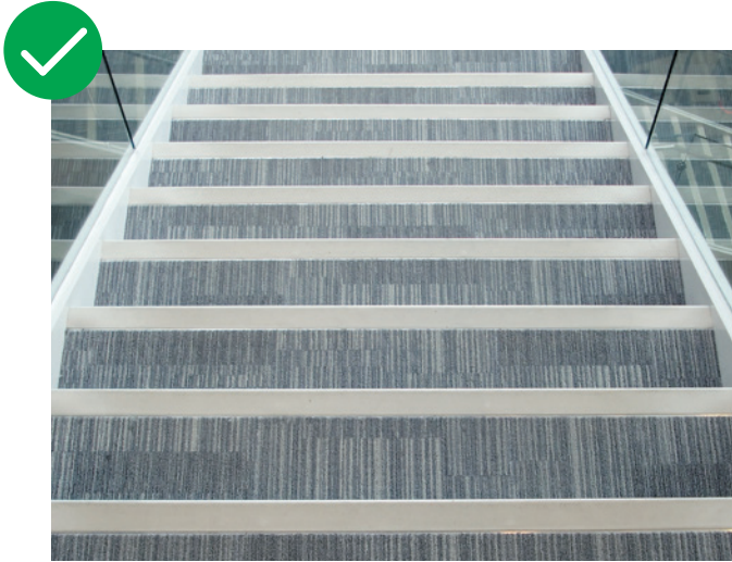
Good Visual Contrast Installed with Gradus Stair Nosings
