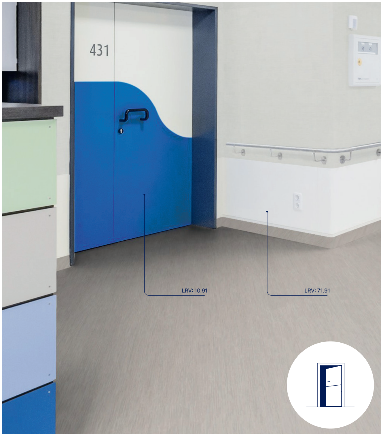
Image shows more than 30 LRV points between the door and wall – Patient door
