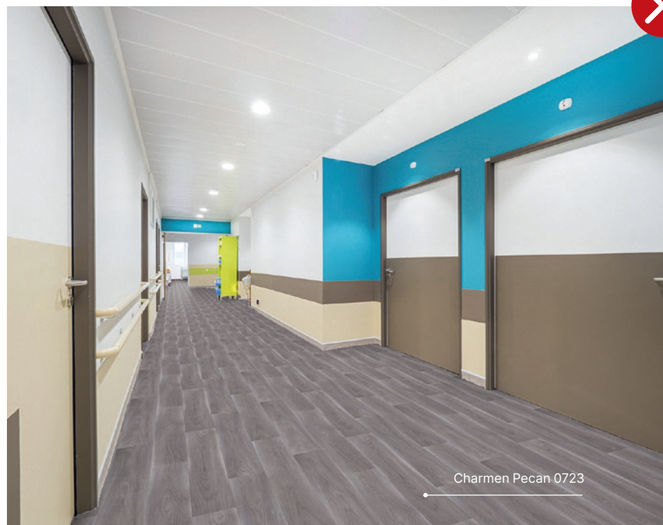
Example of a contrasting floor design which could be perceived as undulations
