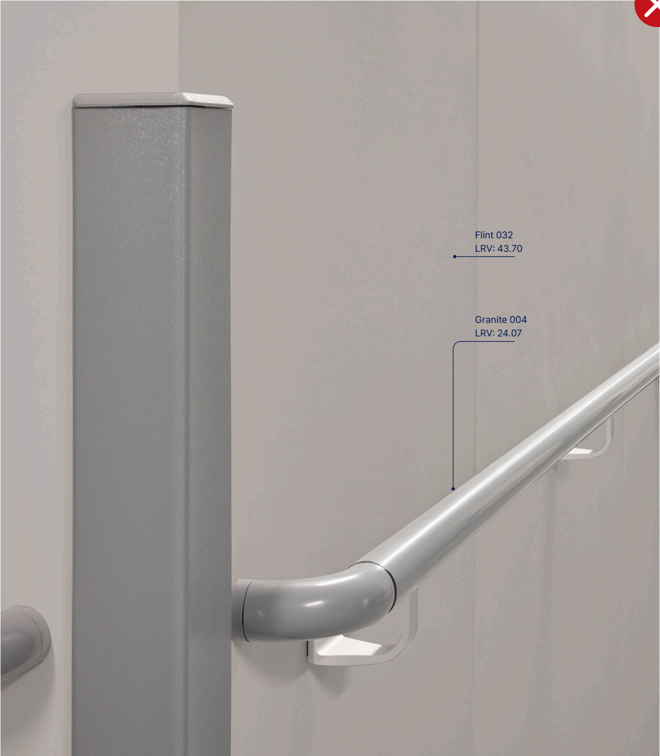
Image shows less than 30 LRV points difference between the handrail and wall
